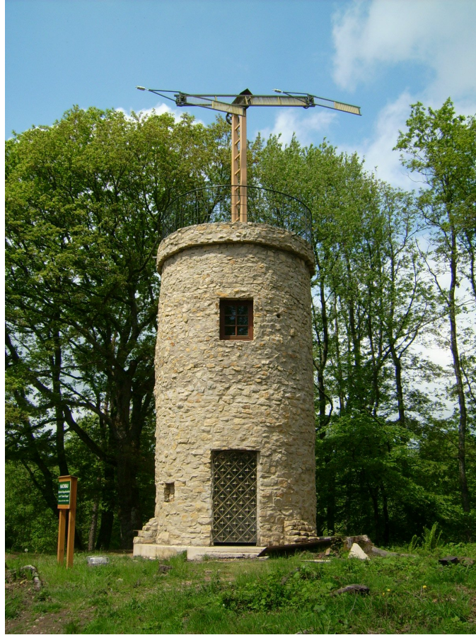
Figure 1.1 Chappé telegraph station near Nalbach, Germany [85]
